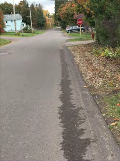
East 7th Ave. facing west
