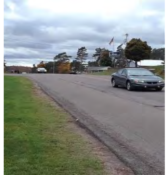
No separation of shoulder from the road. Cars are also moving faster than the speed limit.
