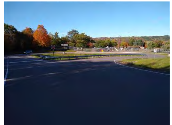
Shortcut through parking lot maybe dangerous as there is no painted crosswalk.
