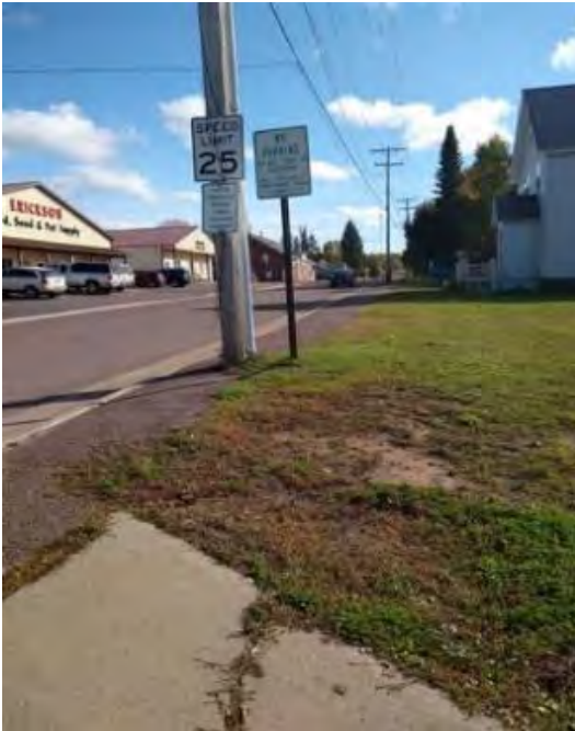
Street is too narrow and there is little distinction between the road and the sidewalk. Cars have low visibility when turning.
