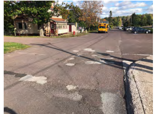
Jacker Ave, facing east
