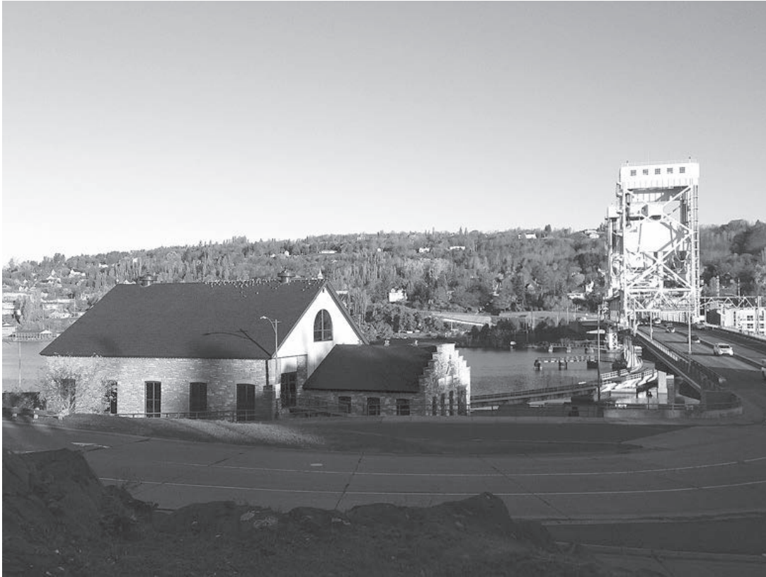
Figure 2. The Powerhouse, Houghton, Mich. (Photo by John Arnold)
